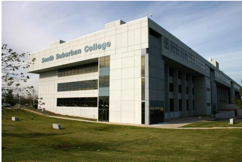
The South Suburban College main campus in South Holland, Illinois.
